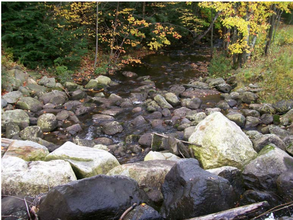
Photo 22 - Downstream channel viewed from the spillway crest.
