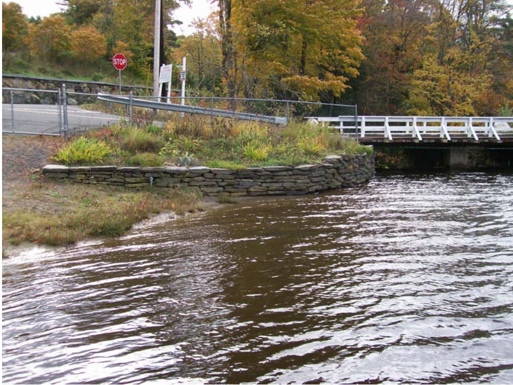
Photo 13 - Upstream view at Left abutment.
