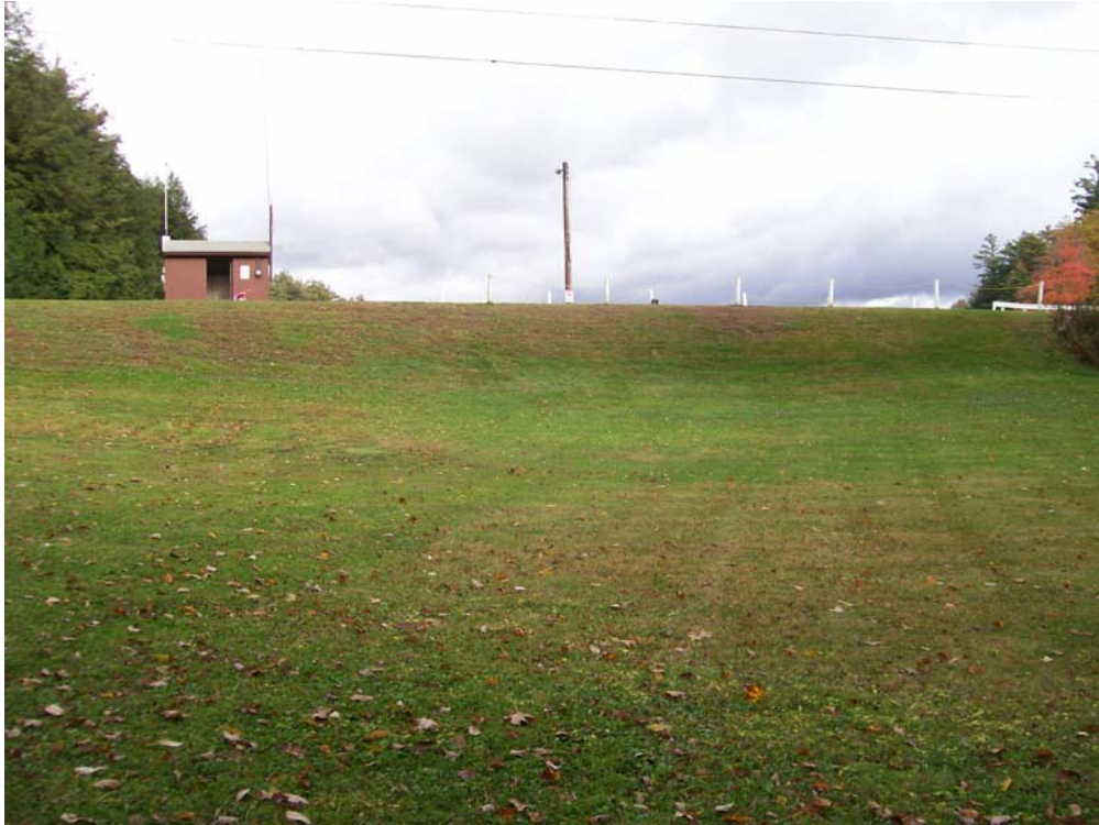
Photo 3 - Downstream slope viewed from downstream center.
