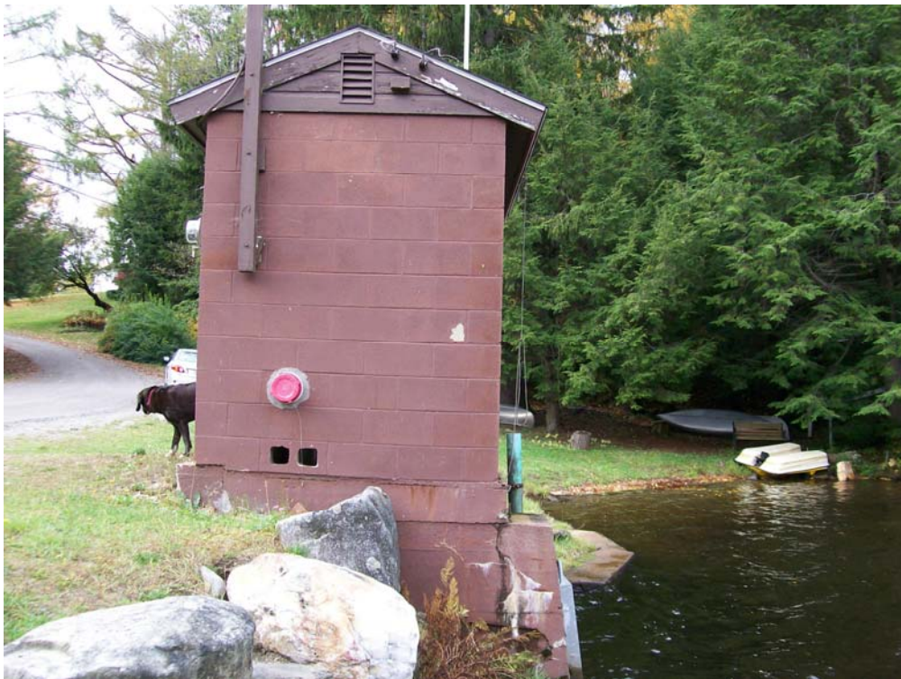
Photo 16 - Gatehouse viewed from left side.
