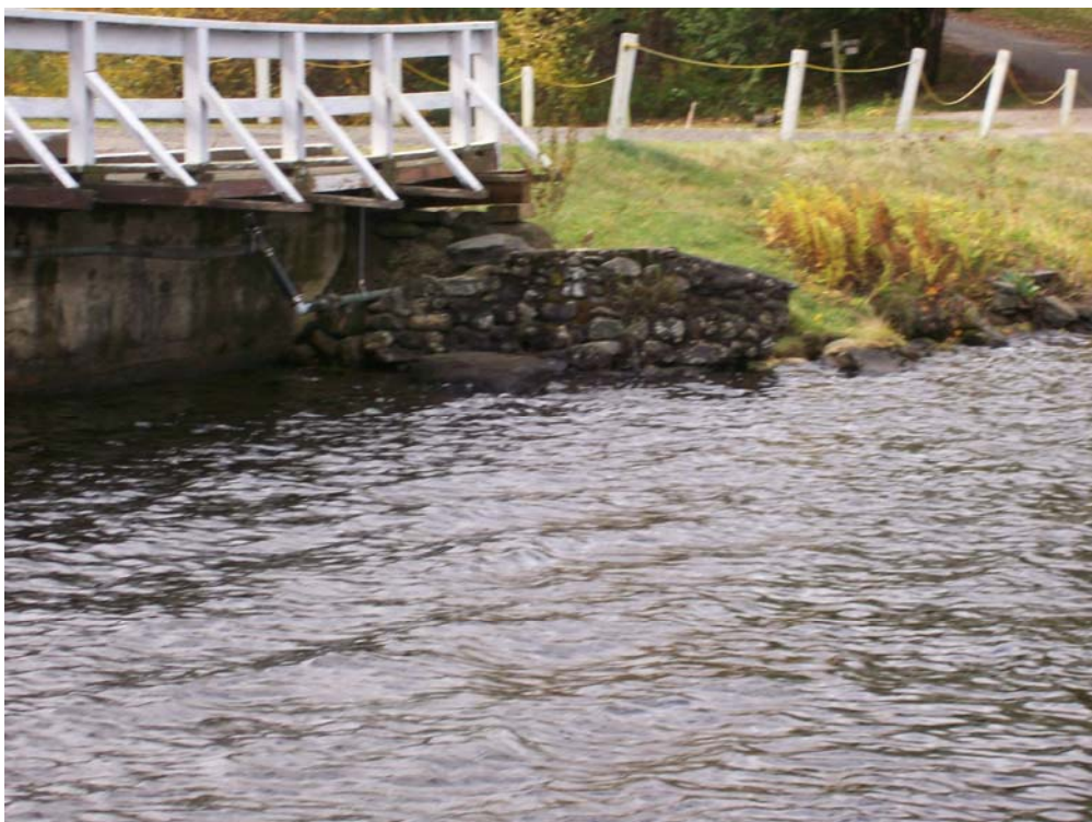
Photo 20 - Stone masonry training wall at upstream right side of spillway.
