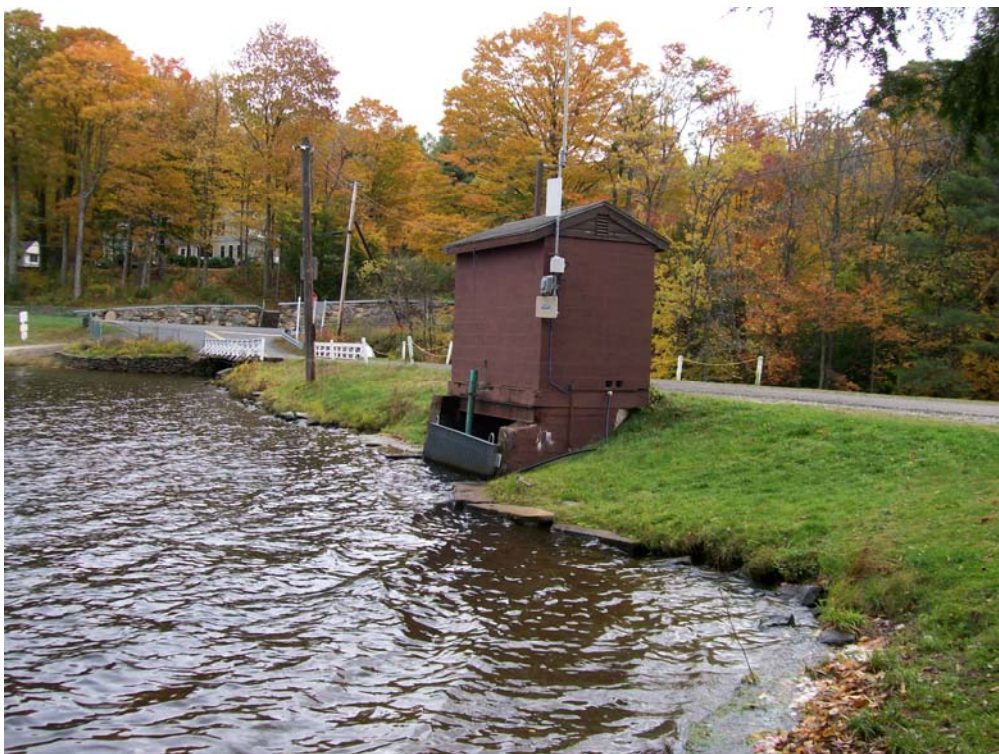
Photo 2 – Upstream overview of dam from the right side.
