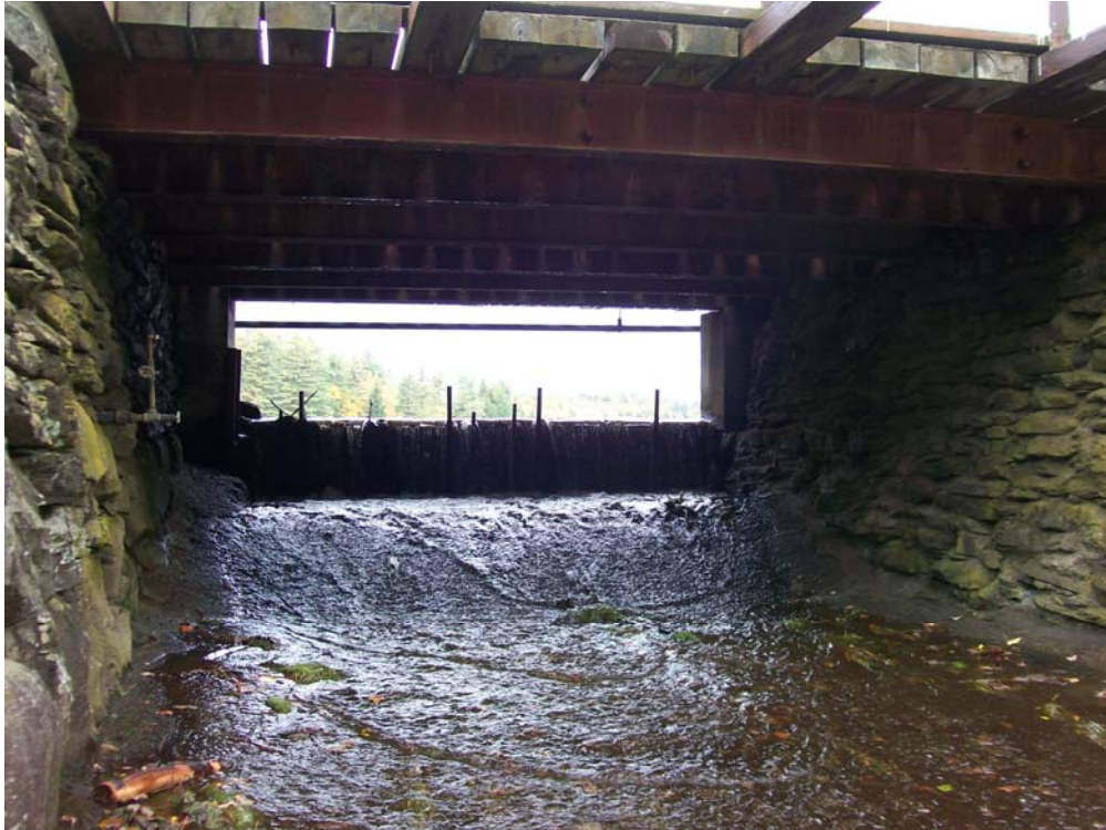
Photo 9 - Downstream view of spillway's right bay.
