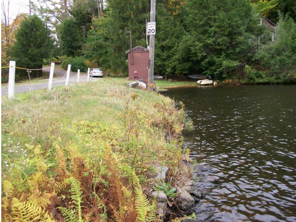
Photo 15 - Stone masonry and rip rap along lower portion of upstream slope.
