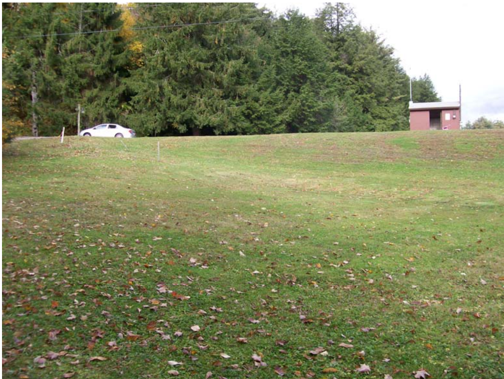
Photo 4 - Downstream slope at right abutment.
