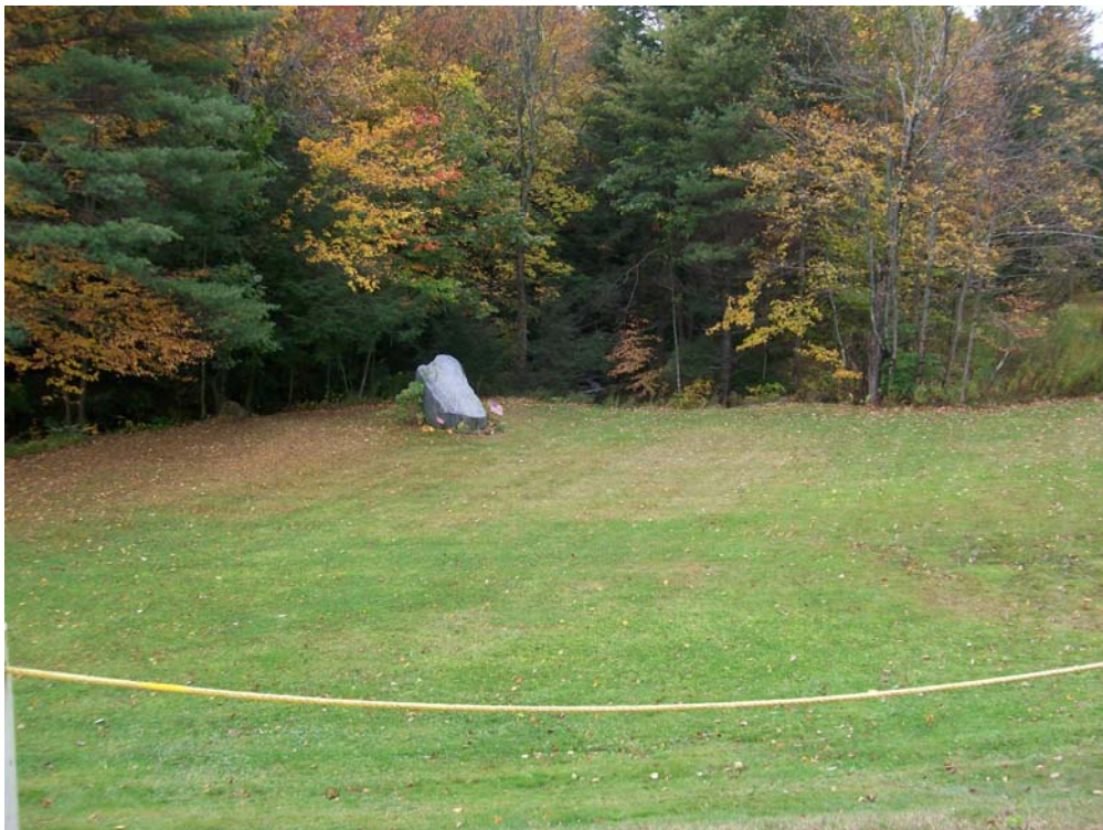
Photo 6 – Downstream area viewed from dam crest at center of dam.
