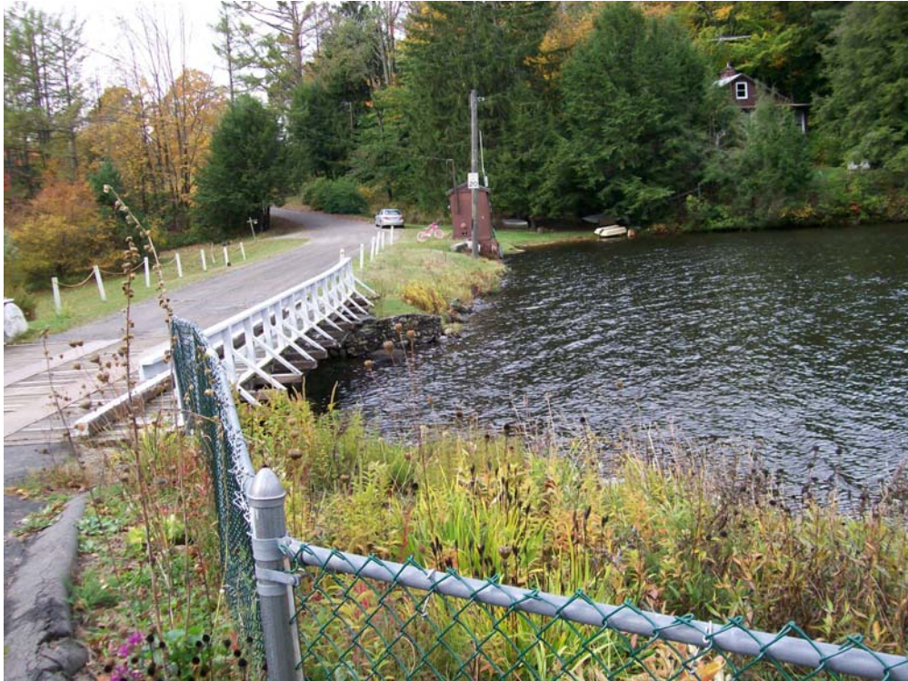
Photo 1 – Upstream overview of dam from the left side.
