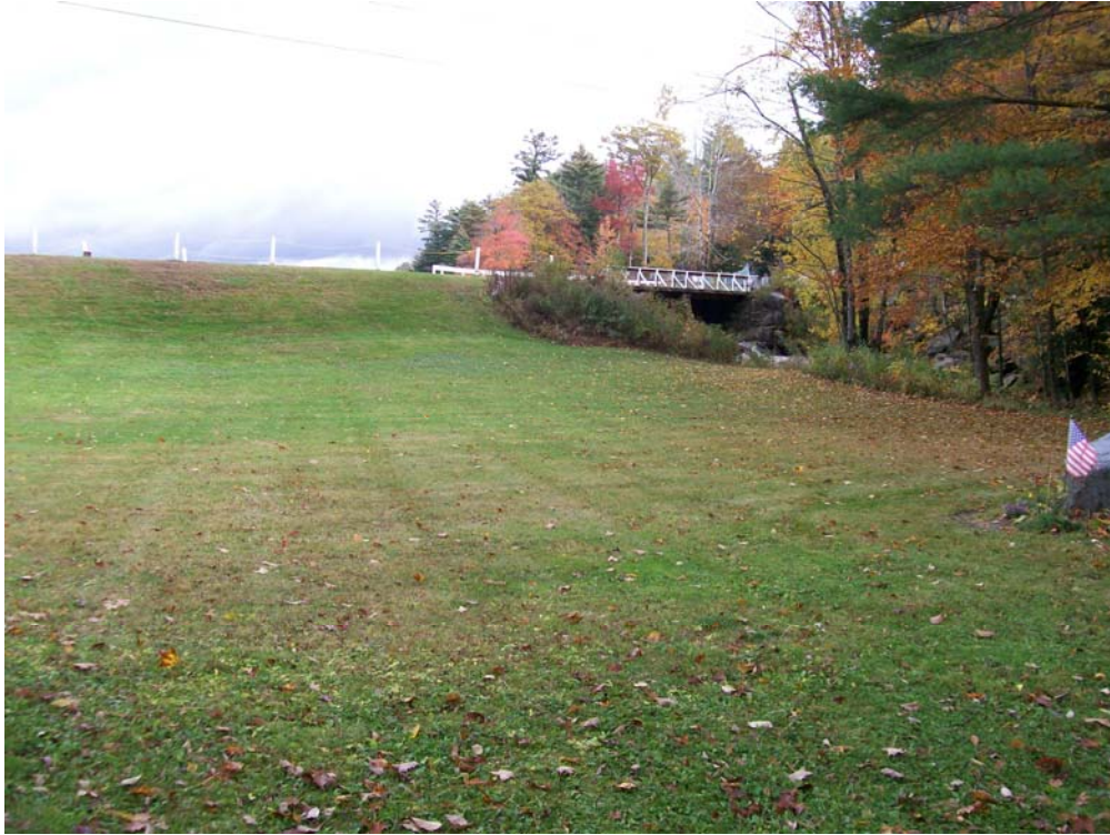
Photo 5 - Downstream slope and spillway at left abutment.
