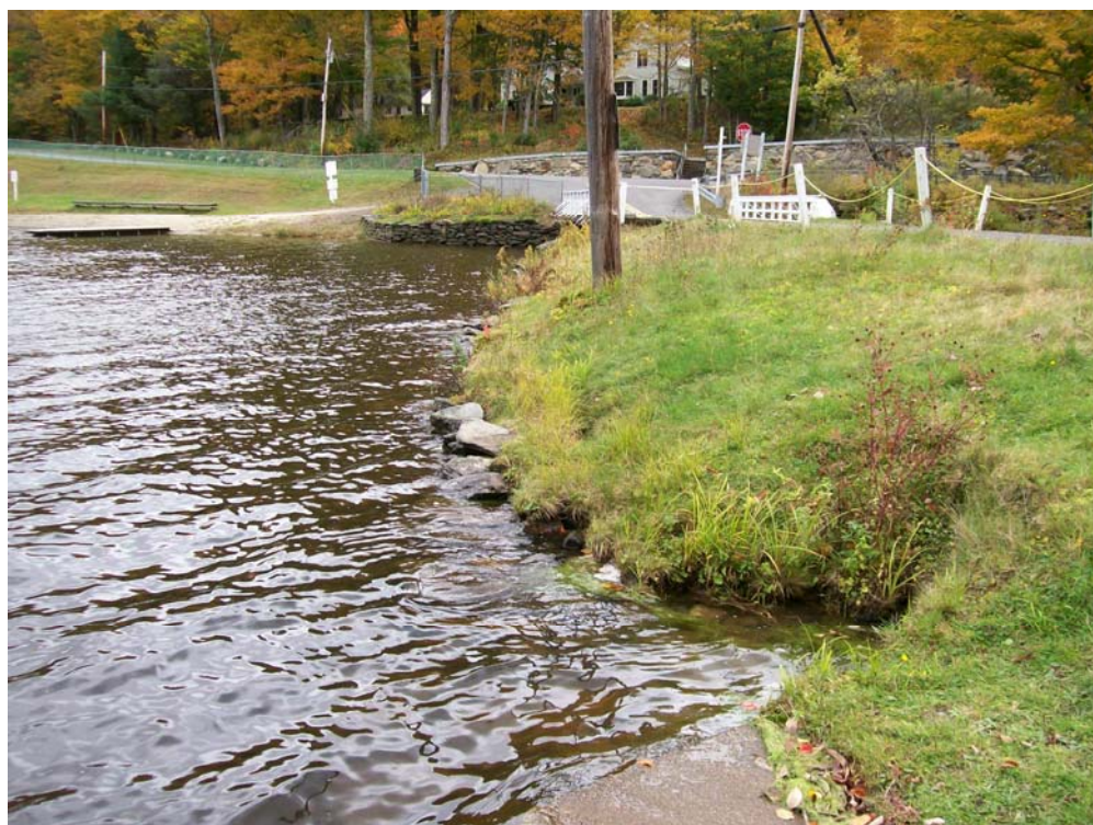
Photo 18 - Rip rap on upstream slope, viewed from the right side.
