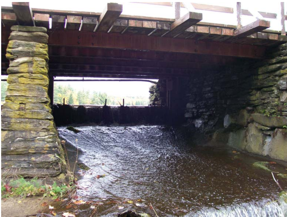
Photo 10 - Downstream view of spillway's left bay.
