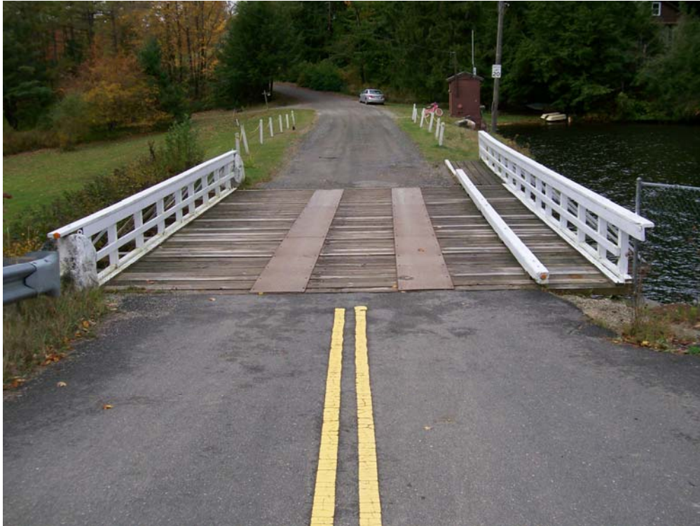
Photo 7 - Dam crest viewed from the left abutment.
