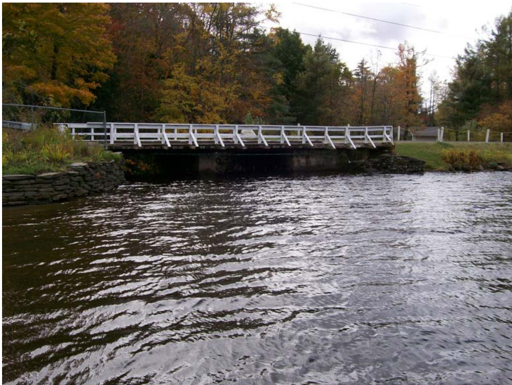
Photo 14 - Upstream view of spillway.
