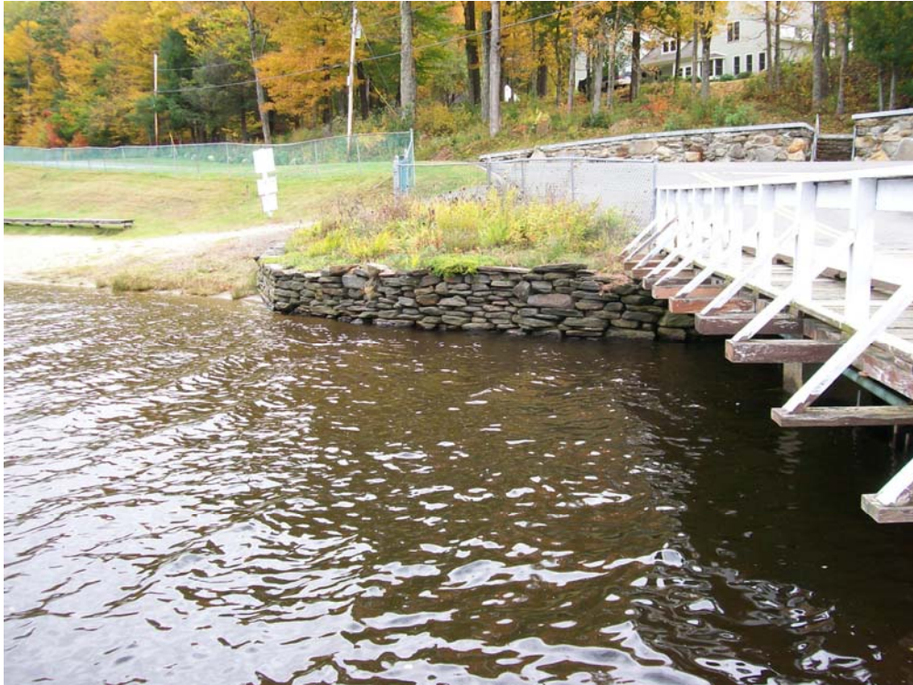
Photo 19 - Field stone masonry training wall at upstream left side of spillway.
